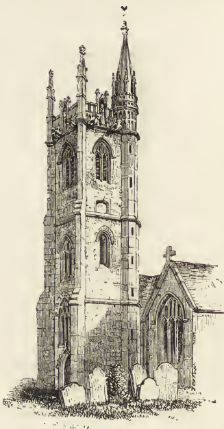
156. Brislington, Somersetshire, c. 1500.
